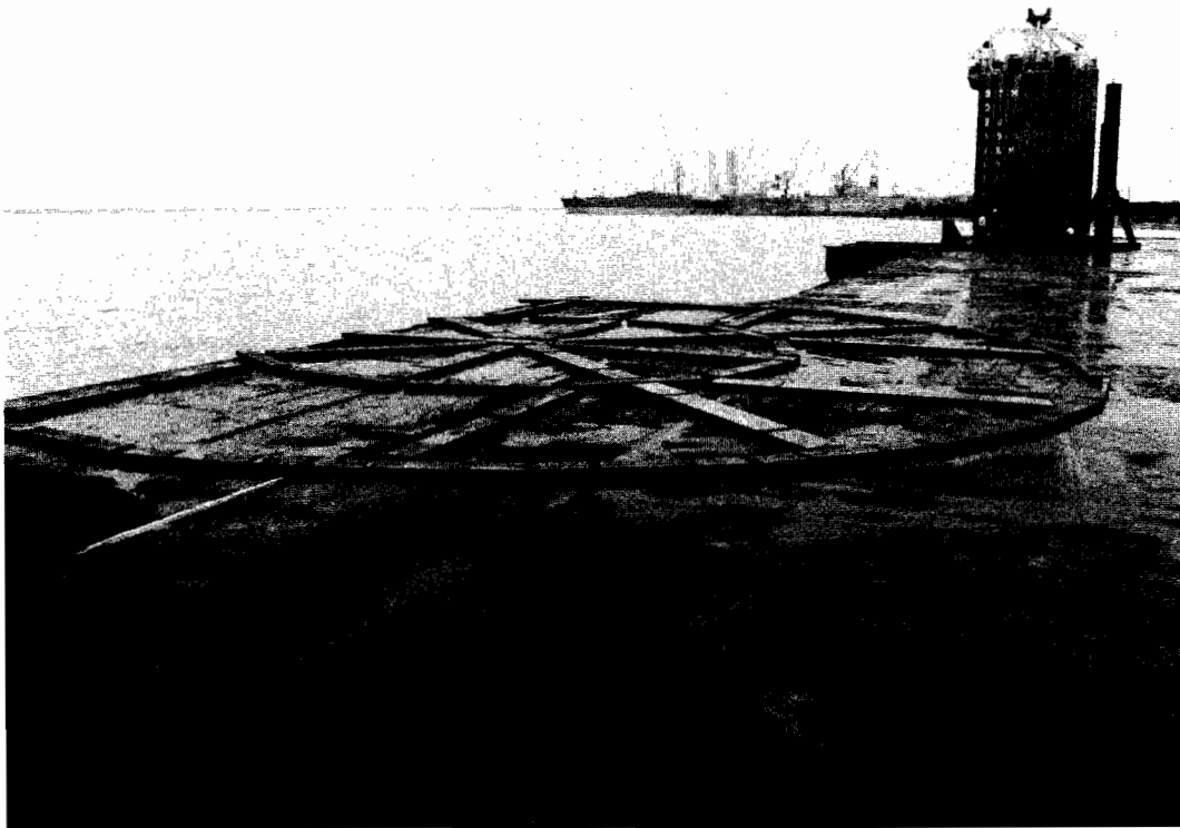
Fig. 10 - Cribbing arrangement for forward starboard column.
