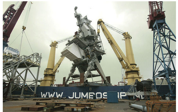
Figure 3 Fairpartner lifts and loads a 1,800 t heavy J-Lay tower [4]
